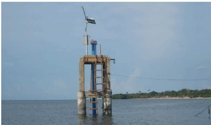
The newly established Lubang Tsunami Warning/Sea Level Station located at Lubang Island, Occidental Mindoro. Established in June 2010, it is an offshore platform installation funded by the UN Economic and Social Commission for Asia and the Pacific, facilitated by ADPC/RIMES, and assisted by NAMRIA oceanographers.
